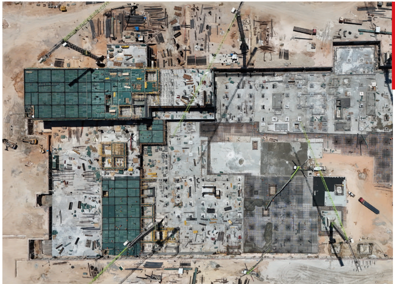
PHOTO COURTESY OF PEKERLER INSAAT ARCHIVE
