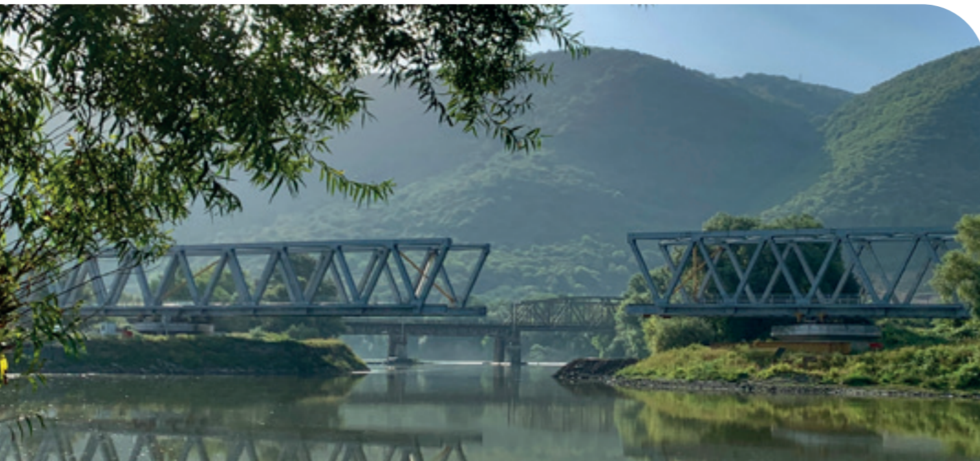
Mures Railway Bridge - Romania
