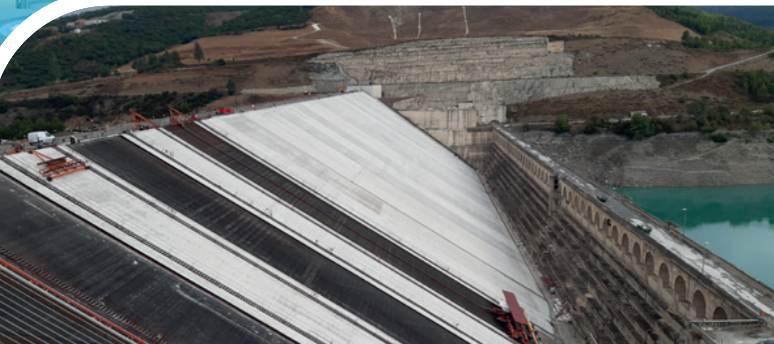
Yesa Reservoir - Spain
