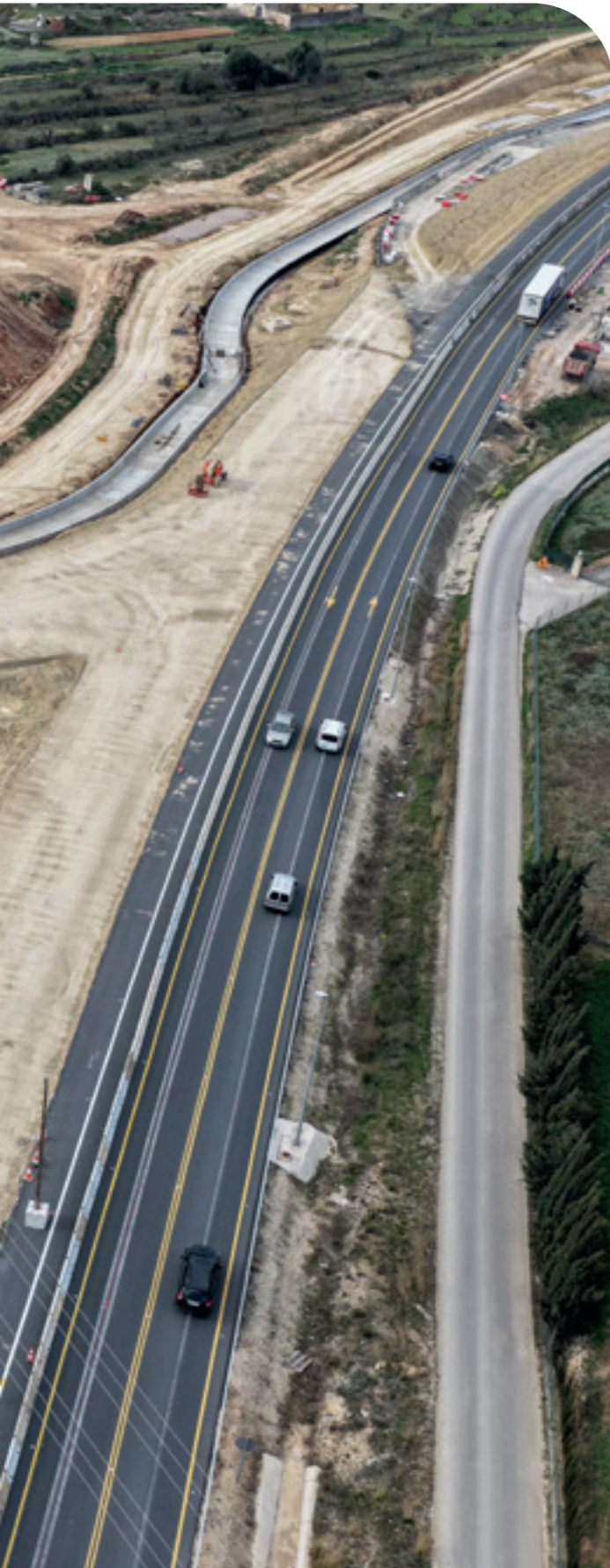
Benissa Bypass - Spain
