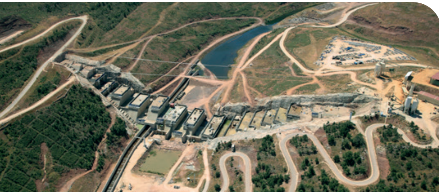
Castrovido Dam - Spain
