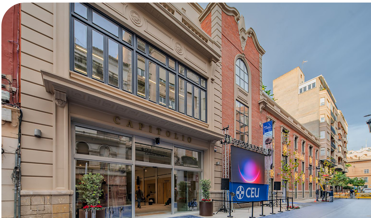
Rehabilitation of San Pablo CEU University, Valencia – Spain
