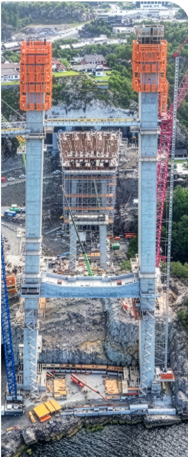
Sotra Bridge – Norway
