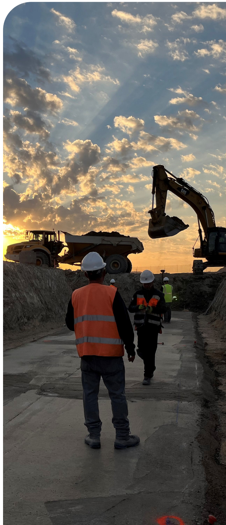
Berrocales Residential Development – Madrid – Spain
