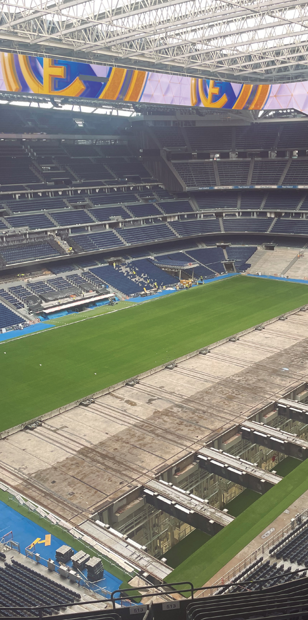
Remodelling of the Santiago Bernabéu stadium (Madrid, Spain)
