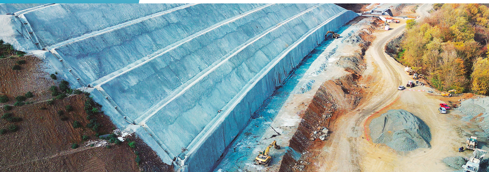
Construction of different railway sections (Romania)
