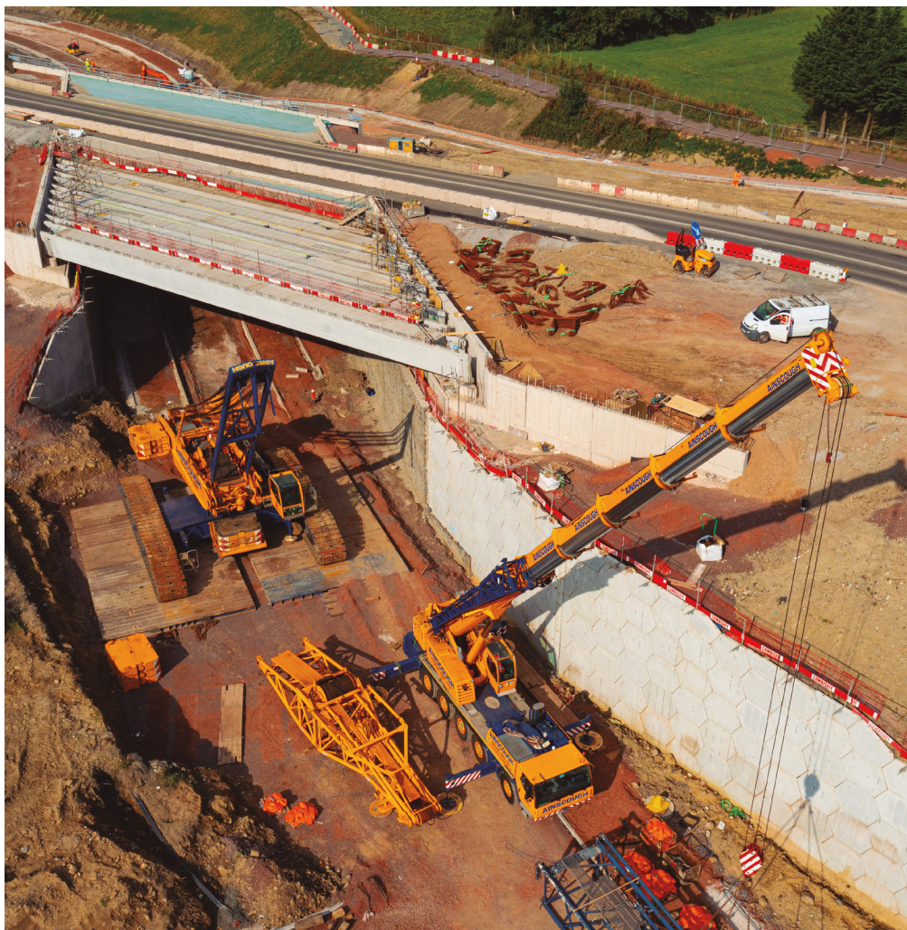
Expansion of the A-465 dual carriageway, sections 5 and 6 (Wales, UK)
