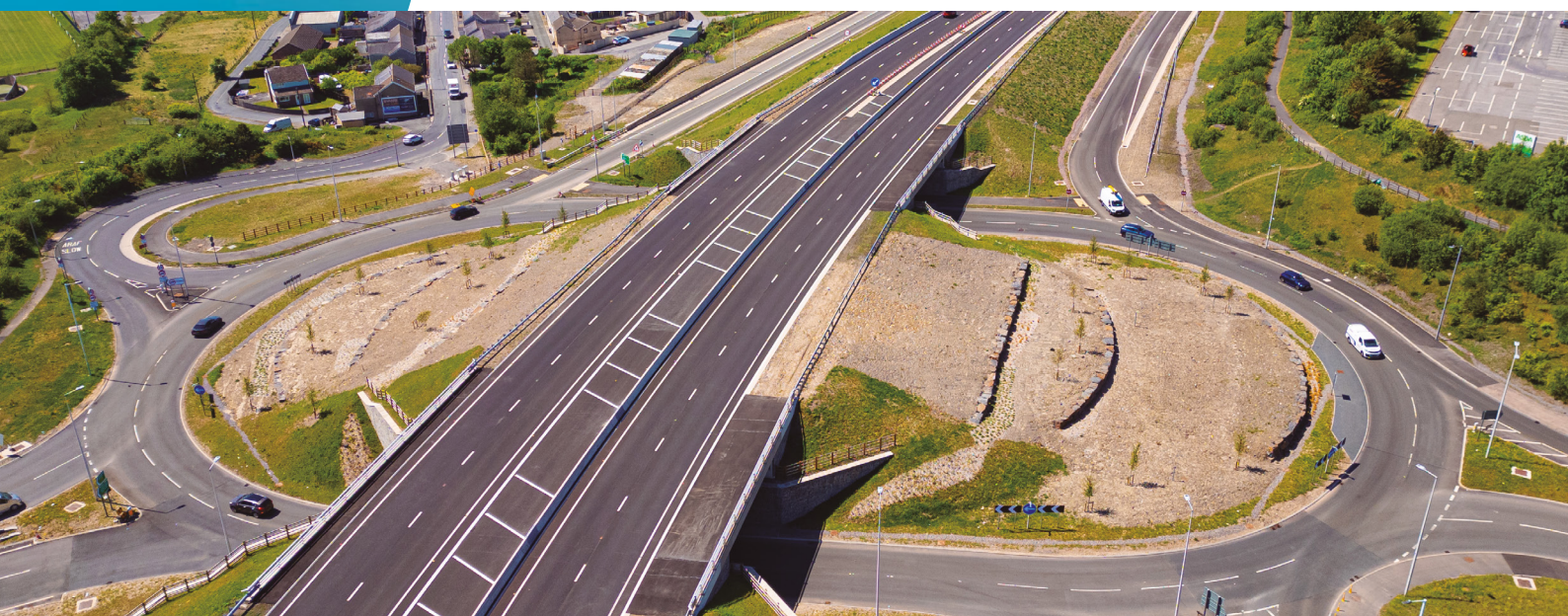
Widening of the A-465 dual carriageway, sections 5 and 6 (Wales, UK)
