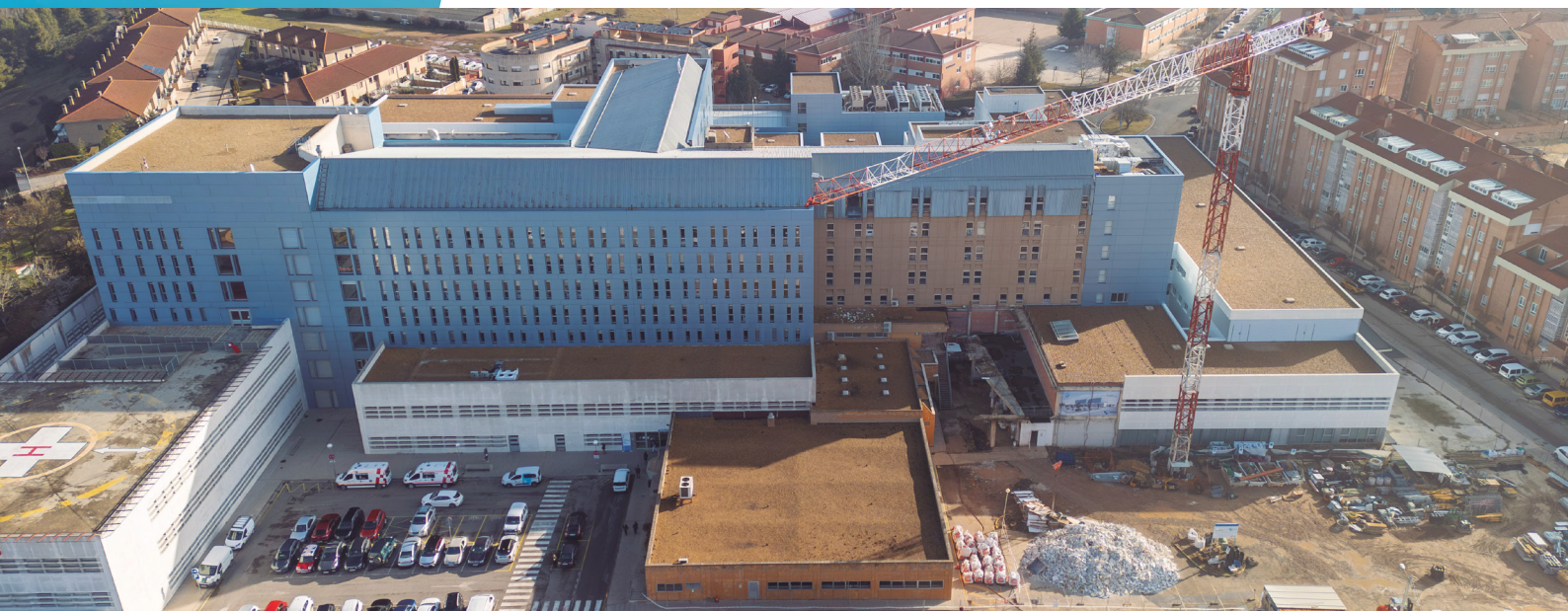
Expansion of the Soria Hospital (Spain)
