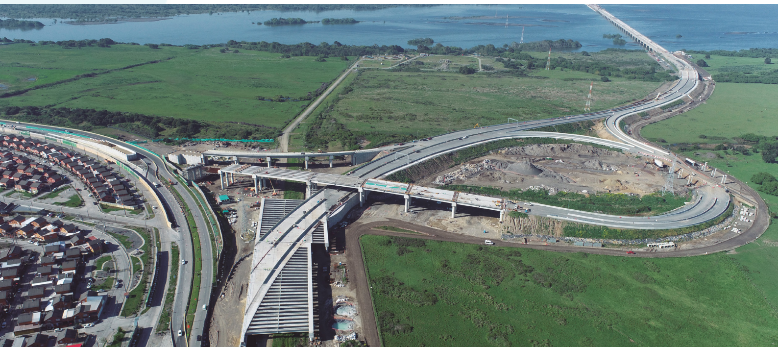
Industrial Bridge (Chile)
