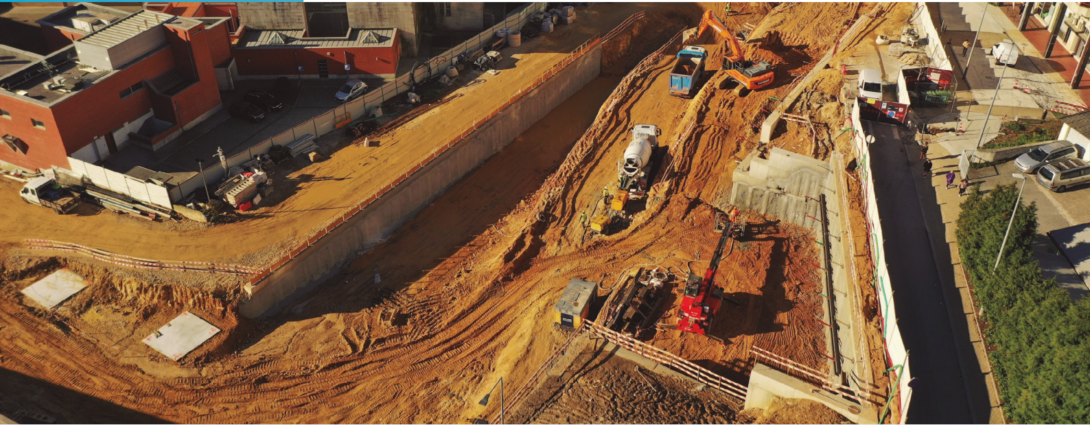
Expansion of the Oporto Metro line (Portugal)
