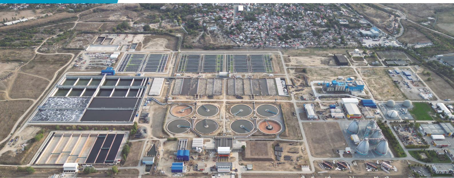
Glina wastewater treatment plant (Romania)
