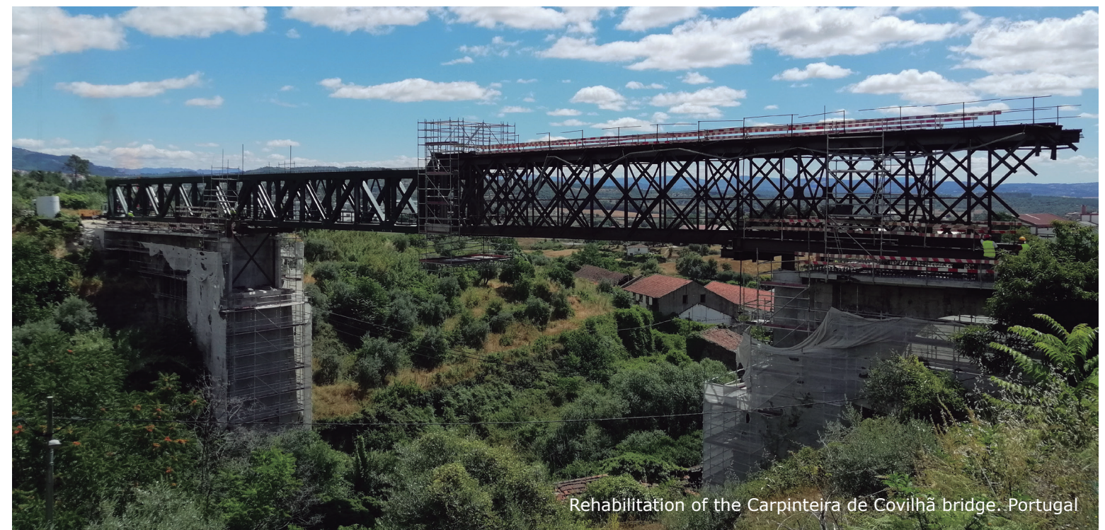
FCC Construcción Verified Emissions Report 2021
