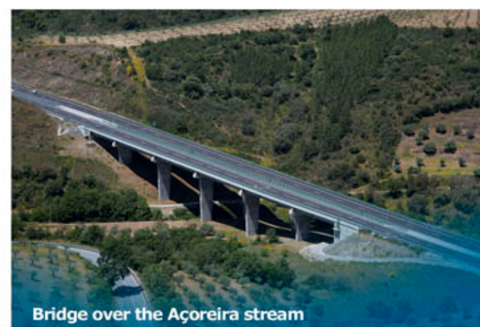
Bridge over the Açoreira stream
