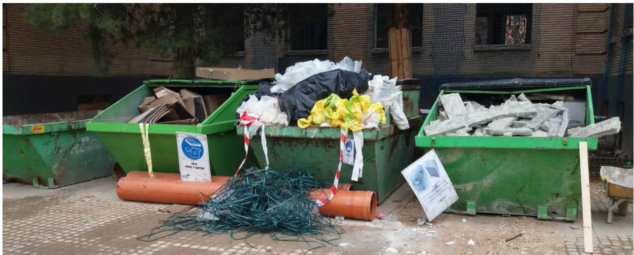
Distribution of containers in order to carry out proper waste segregation in the remodelling works at the University of Zaragoza.
