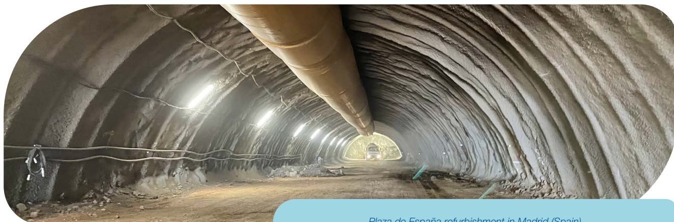
Plaza de España refurbishment in Madrid (Spain)
