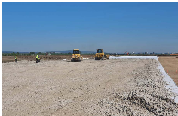
Reuse of waste on the new runway and taxiways once they have been shredded.
