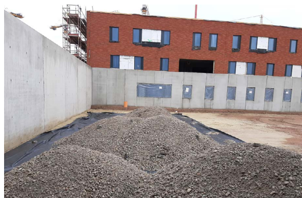
Aggregate arranged to be spread out in the courtyard outside the prison.
