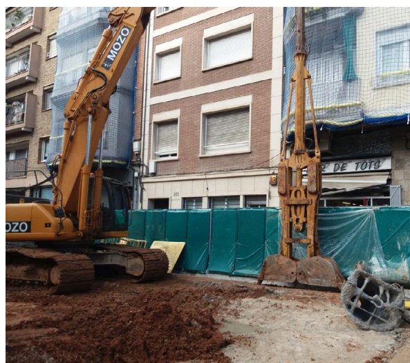
Overview of the soundproofing panels on site. Maragall Metro Station (Barcelona).
