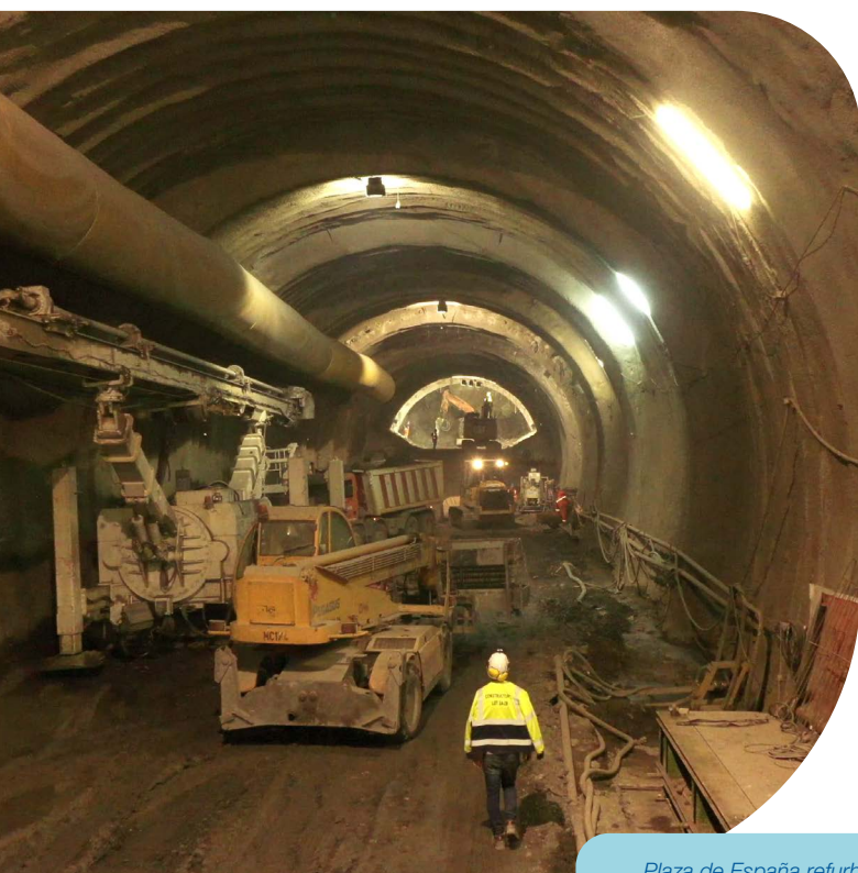
Plaza de España refurbishment in Madrid (Spain)
