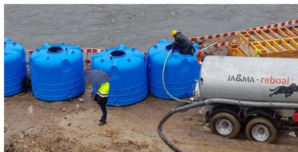
Tanker truck on site to be able to take contaminated water to the existing treatment system at a nearby construction site, if necessary.
