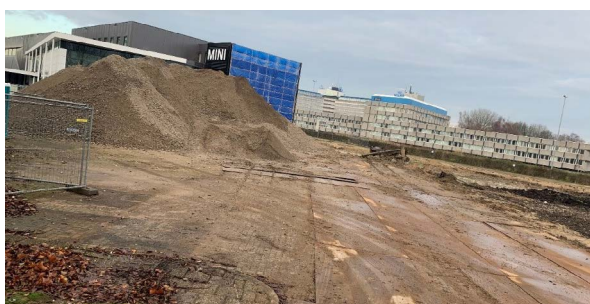
Stockpiling materials after crushing for later reuse.
