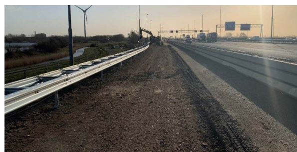
Spread of recycled material on the A9.
