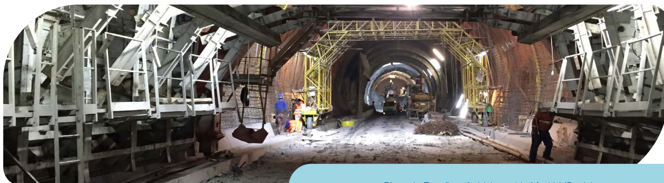
Plaza de España refurbishment in Madrid (Spain)
