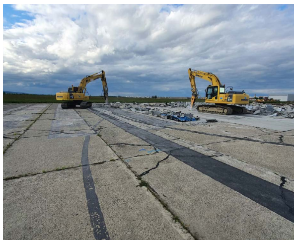
Demolition of the Bacau airport runway.
