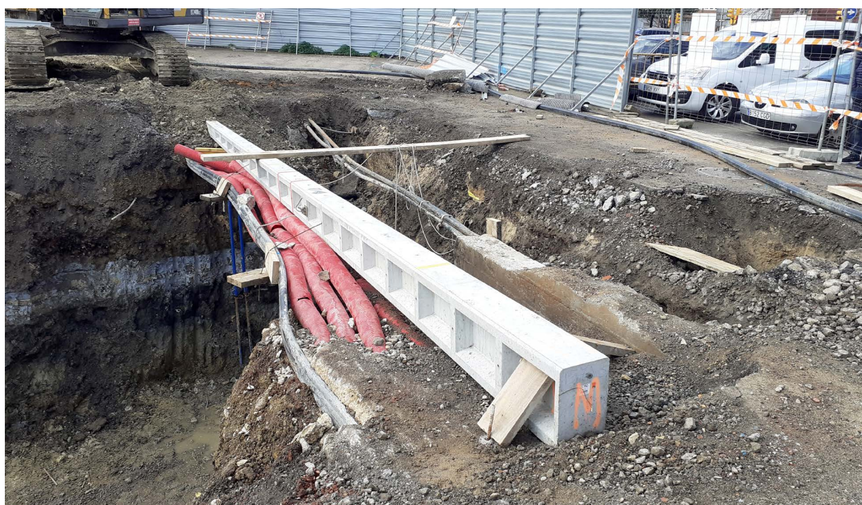
Detail of the temporary shoring of these services for their protection.
