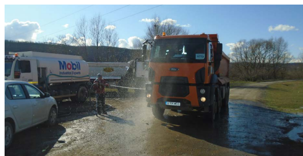
Cleaning of trucks at the site exit to reduce dust emissions in the project environment.
