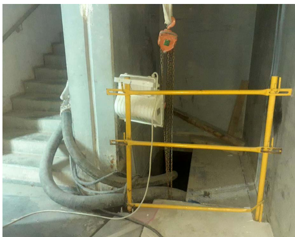
Pipes direct water through the shaft levels to ground level.
