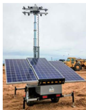
Hybrid lighting tower on the construction site of the new runway at Dublin Airport.
