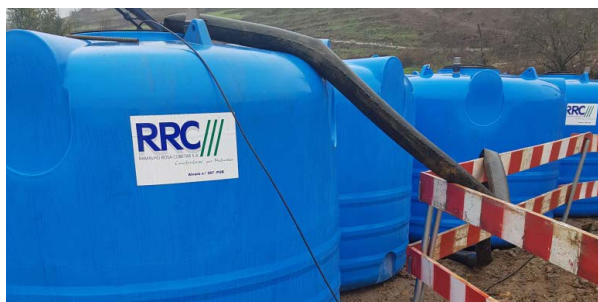
Tanks for pH control of the influent water from the water table that comes into contact with the fresh concrete.
