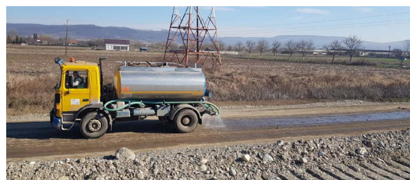
Watering of roads to reduce dust emissions caused by vehicle traffic during the transport of materials or people.
