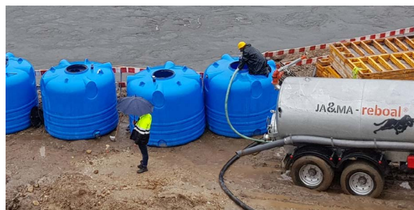
Tanker truck on site to be able to take contaminated water to the existing treatment system at a nearby construction site, if necessary.
