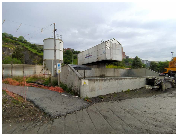
View of the decanter, filter press and treated water tank. The coagulation and flocculation processes, as well as the settling and clarification processes, allow the removal of suspended solids dissolved in the water. Subsequently, pH adjustment is carried out prior to discharge.
