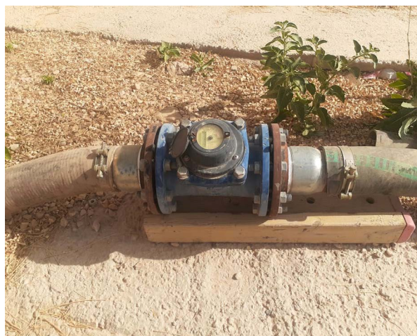
Water meter installed by the municipality of Riyadh to monitor the amount of water used.
