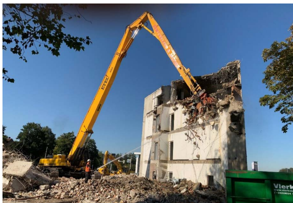
Selective extraction and separation of waste for subsequent recycling.
