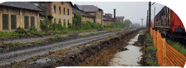
Detail of the contaminated soil surface that was removed for the application of bioremediation techniques at the Simeria station
