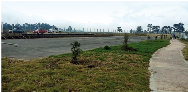
Building of Parque San Nicolás.
