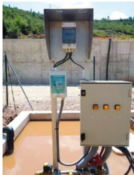
Control unit for monitoring pH, regulating influx of CO 2 and catchment pool for subsequent treatment with CO 2 .
