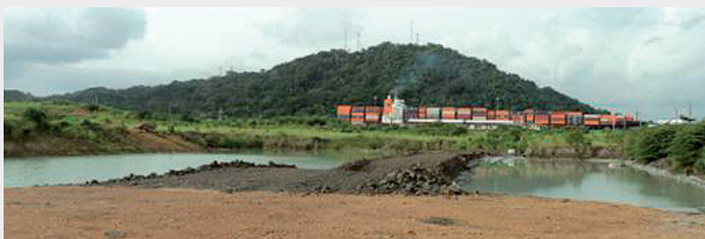
Division of the pool - the central dyke acts as a filter.
