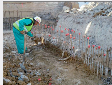
Cleaning the mud mixed with bentonite from the adjacent screen walls.
