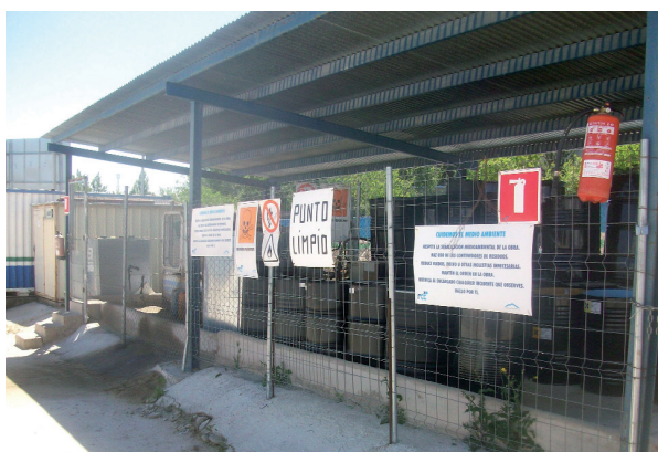
► The containers for the storage of hazardous substances and waste must be clearly identified with the appropriate symbol and label.
