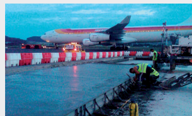
Laying the HP45 slabs.
