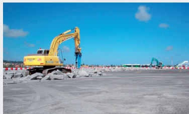
Demolishing the apron concrete slabs.
