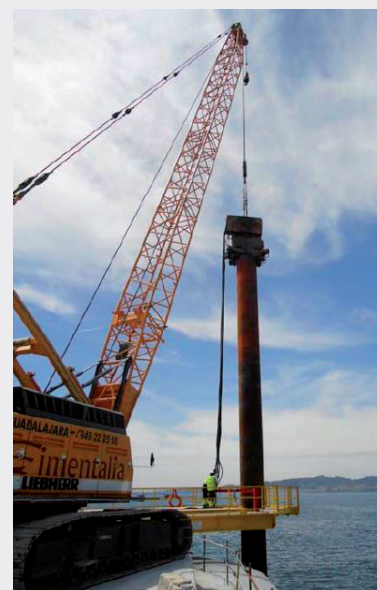
A hydraulic vibrohammer in action driving lost casings.
