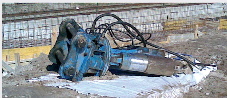
Protection of the ground on which equipment and machinery are parked.
