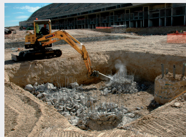
The initial project involved digging a trench for each pile head, which made the pile head stripping and steelwork tasks, and the formwork for them more difficult.
