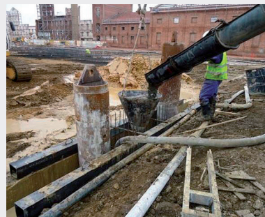
Placing the tubes before concreting the slurry wall.
