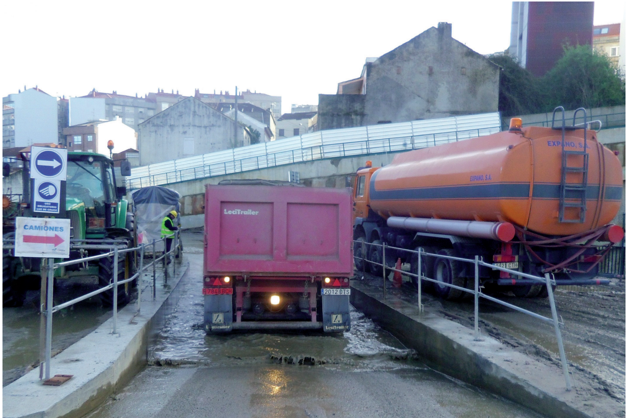
➤ Washing the wheels of trucks before they reach the public highway prevents mud and dust from being deposited, which is especially important when the site is located in an urban area.
