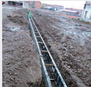
Building the guide wall with formwork on one side.
