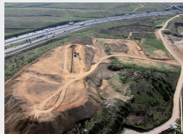
Machinery excavating earth for the foundation landfills.
