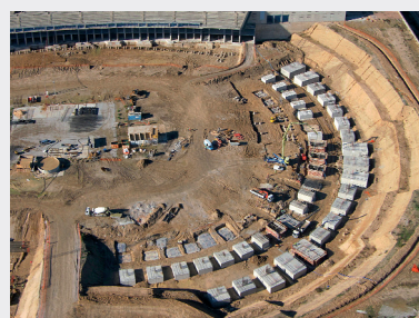
The definitive solution for fitting the foundation pile was to dig a trench to ensure that the work could be executed correctly.
