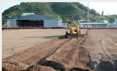
Spreading and levelling crushed concrete fill.
