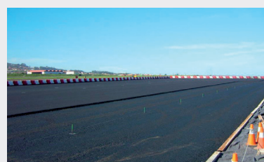
Laying the asphalt agglomerate.
