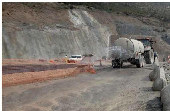
Using both manual and mechanical means, the spraying of the roads and materials supplied becomes a simple and efficient Good Practice in order to reduce dust emissions, mainly associated to earth movement, the vehicle traffic and the transport of earth and rubble.
