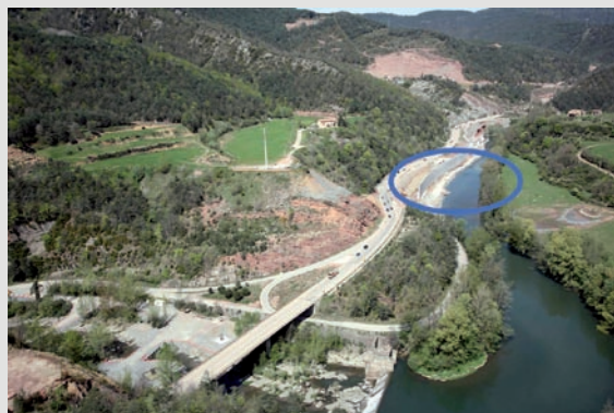
Aerial photograph of the wall under construction and of settling basins aligned in a crescent shape row located on the opposite bank of the River Ter.
