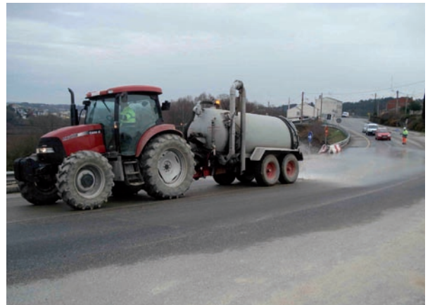
In the event of temporary occupation of roads, it is essential to reduce discomfort for the users. One of the actions taken for this purpose is the systematic cleaning of highways and roads.
