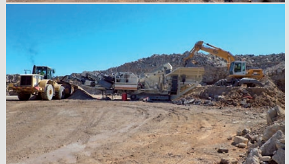
Recycling of CDW onsite.
