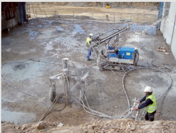
Machine boring for consolidation grouting
