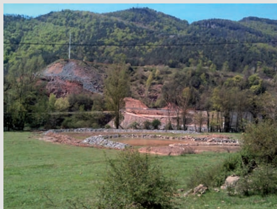
Detailed view of settling basins aligned in a crescent shape row located on the opposite bank of the River Ter.
