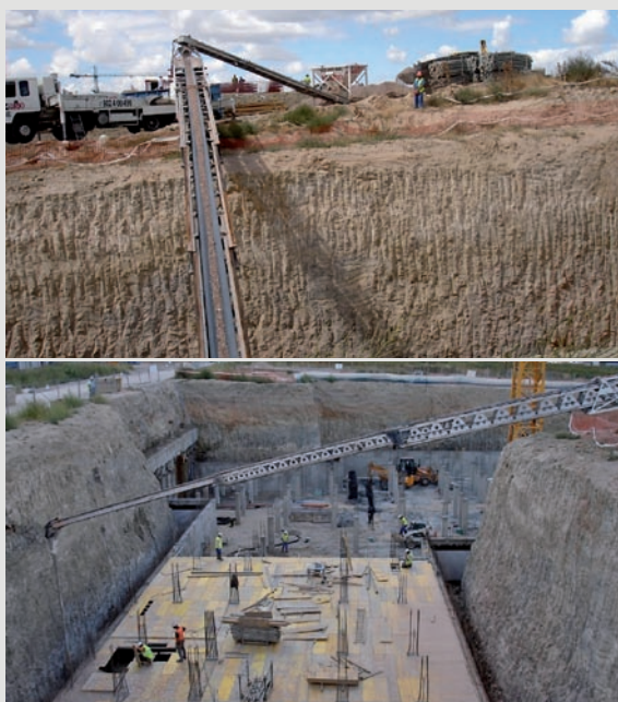
On site placing of the material in basements 2 and 3, using a hoppers conveyor belt in coiled tubing.
