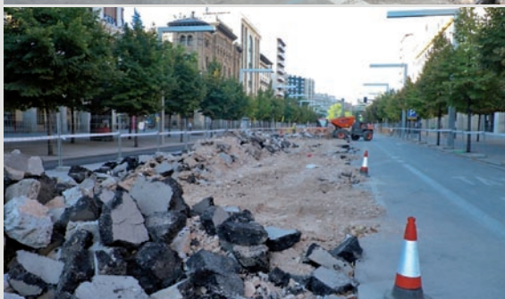
Demolition of the road.
