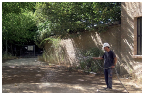
Using both manual and mechanical means, the spraying of the roads and materials supplied becomes a simple and efficient Good Practice in order to reduce dust emissions, mainly associated to earth movement, the vehicle traffic and the transport of earth and rubble.
