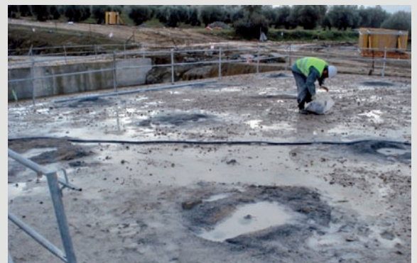
Worker collecting the material after making the boreholes
