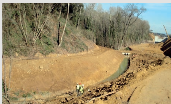
Slope of the new channel.
