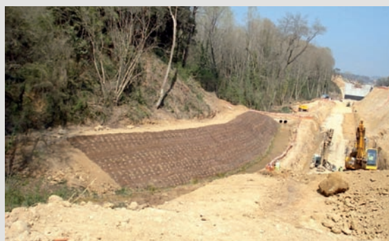
Protecting the slope with geogrids.
