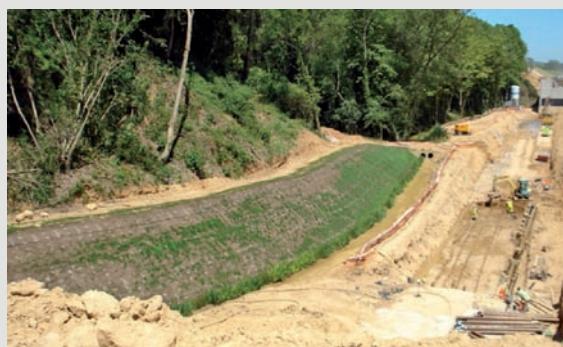
Hydroseeded slope.
