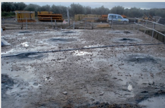
Photograph showing where the dust from the drilling remains once the boreholes are made
