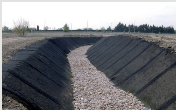
Channelling of the Rejas Stream, with gravel at the channel bottom and slopes upholstered with geogrid hydro-seeded.
