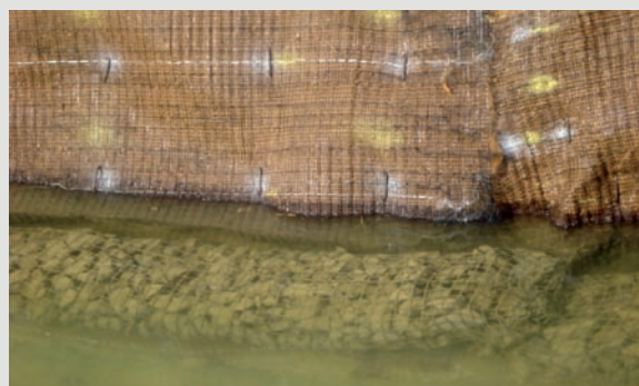
Detail of the gabions and the coconut fibre mat over the geogrid.
