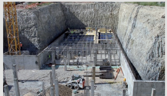
Execution of the basements of dwellings.
