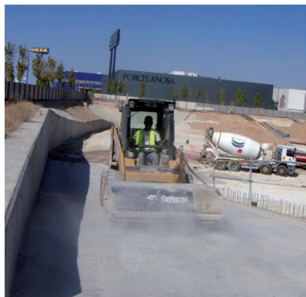
One of the usual methods for avoiding dirt at the entrance and exit of the site is the systematic use of sweeping machines.
