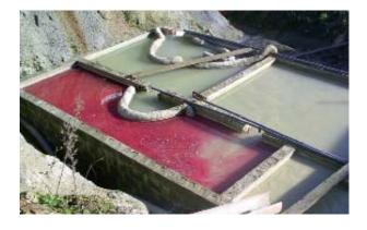
When hydrocarbons are spilled into our settling ponds, we deploy grease and hydrocarbon barriers near the spill to contain it and prevent or hamper it from spreading and moving, and so we limit the size of the polluting event as much as possible. As a complementary measure, we remove these dangerous substances from the pool using absorbent barriers, which float on the water's surface once they have become saturated. Then we place them in appropriate disposal containers and lay out new barriers.
