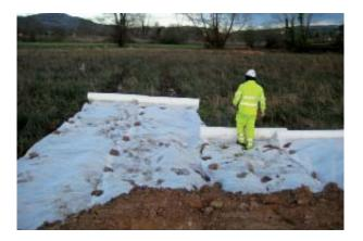
In order to avoid accidental spills of oils, fuels, greases, etc. that might contaminate the soil, impermeable areas are provided where machinery can be greased, maintained and refuelled and tools and machinery can be cleaned.
