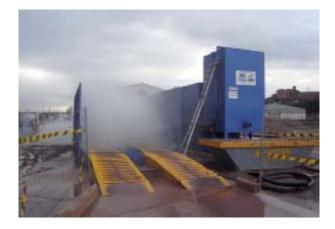
Permanent or mobile systems to wash lorry wheels and undercarriages is a good method for reducing the tracking of mud and dirt onto roads. These low-maintenance facilities clean truck wheels and the resultant sludge is allowed to settle, after which the water is recycled.
