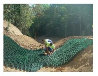
The use of geocells when restoring a water course helps plants to grow back on the banks, because geocells halt erosion and provide plants with pockets in which to take root.
