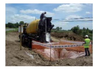
We are aware that water is a very scarce resource that we must use rationally. In many of our projects, we store the water used to rinse out concrete-pouring chutes in properly waterproofed ponds for subsequent reuse.
