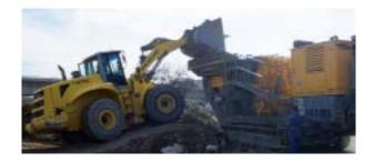
When we find we have a considerable volume of demolition debris on site, we endeavour to recover the rubble. For instance, we can recycle it into aggregate that we can use on site.
