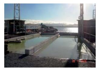
Settling ponds achieve two goals: sedimentation, where the solids in suspension in the water from the project's different activities settle out, and minimisation of the risk of spillage of pollutants and dangerous substances.
