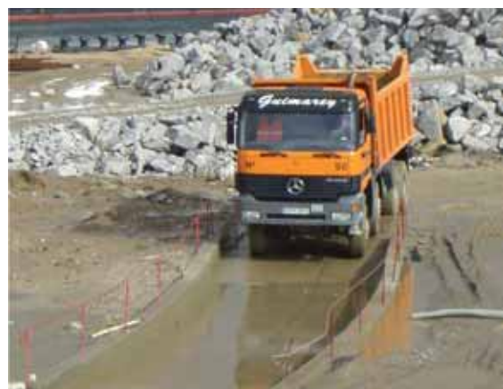
To prevent dirt at the site entrance and exit, it is usual practice to clean the vehicles' wheels before they join the public road.
