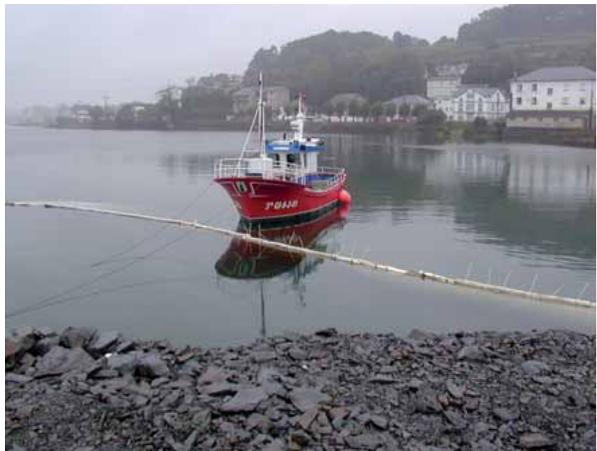
The use of geotextile screens is a very effective method for separating fine matter and, by flotation, oil that could enter the water in emulsion, thus preventing the pollution of nearby water.
