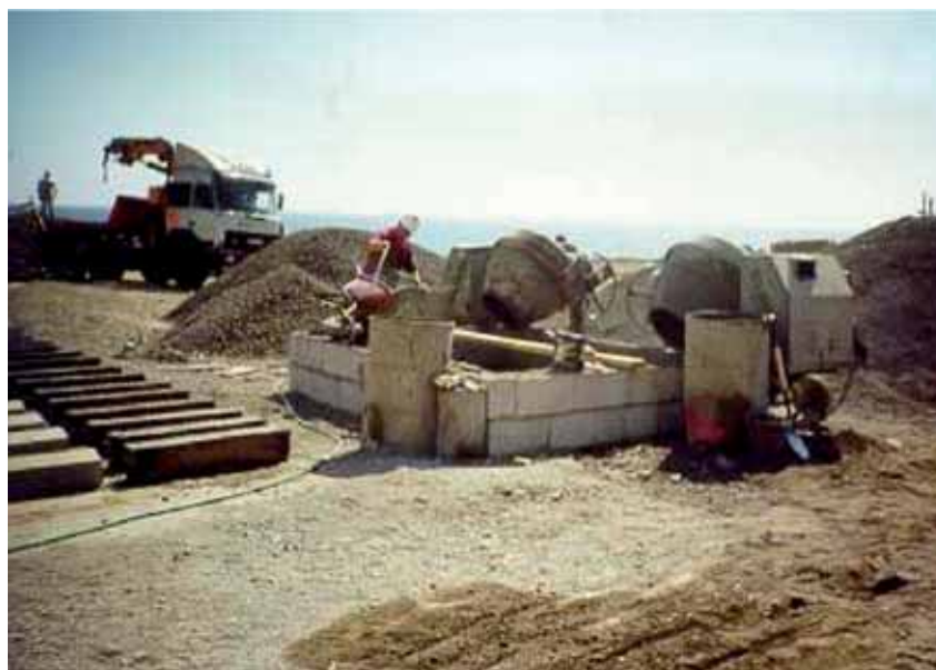
The water from cleaning concrete tubs or other washing has a very basic pH level and must be neutralised before being tipped. An eco-efficient alternative is to use the washing water in the process for manufacturing new concrete, minimising water consumption at the same time.
