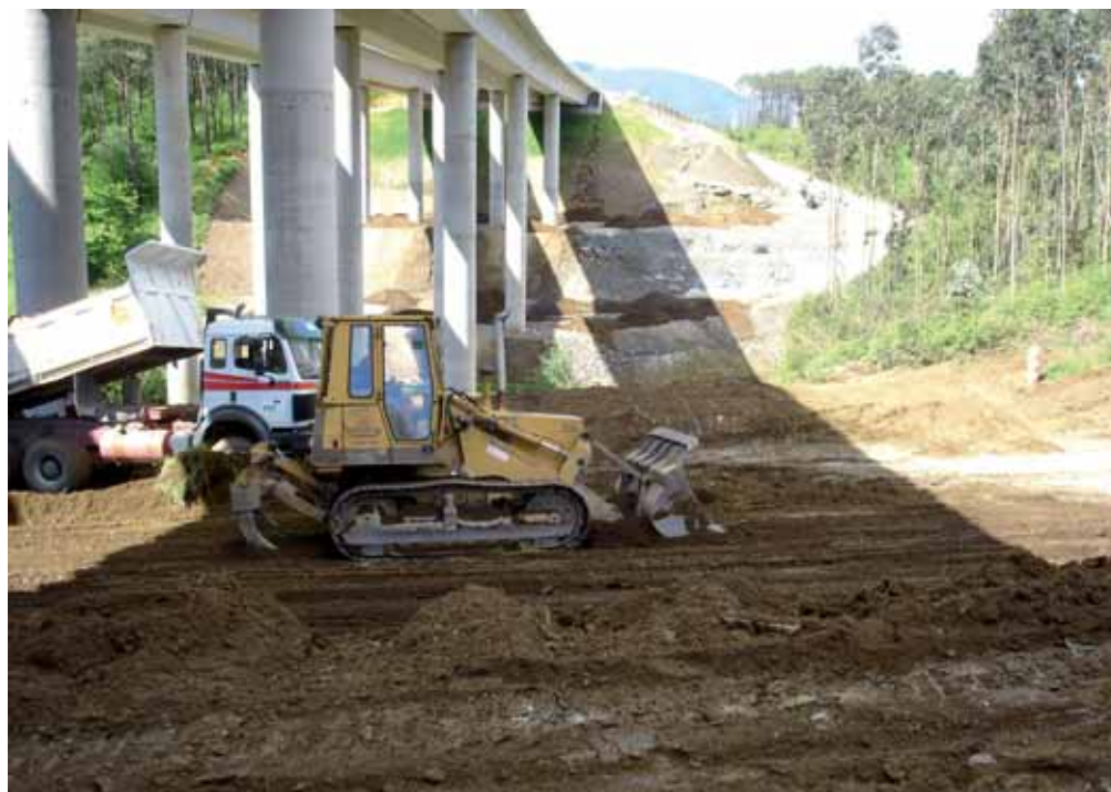
Building involves large movements of soil, requiring suitable planning in order to be able to re-use the earth and gravel extracted on the site, thus reducing financial and environmental costs.
