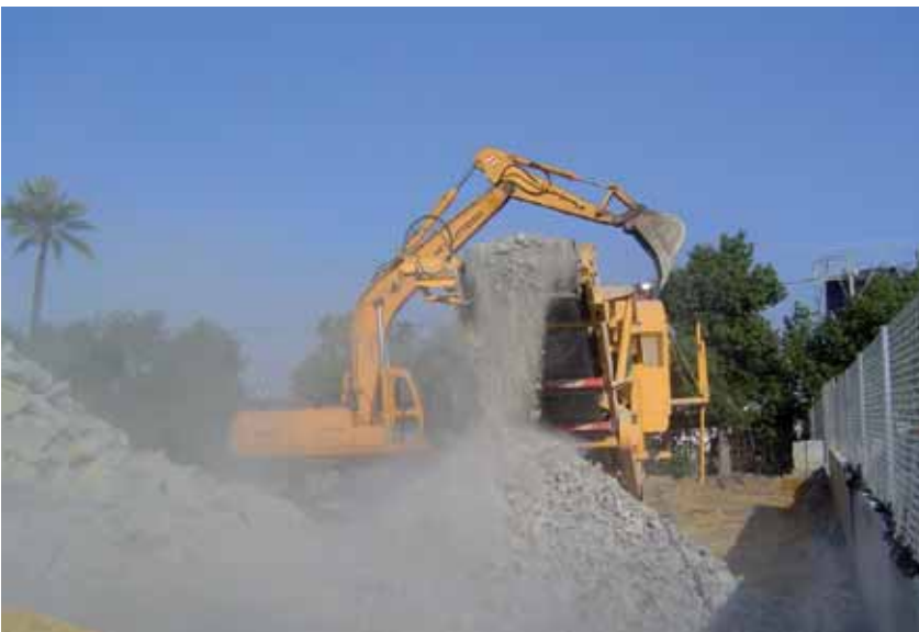
Operations relating to building and civil engineering inevitably generate amounts of dust which we attempt to minimise as far as possible with actions such as spraying the tracks, rubble and stockpiles, reducing the tipping height of material, the use of tubes for pouring rubble from heights, covering the surface of blastings and using screens to prevent the dispersion of dust, among others.
