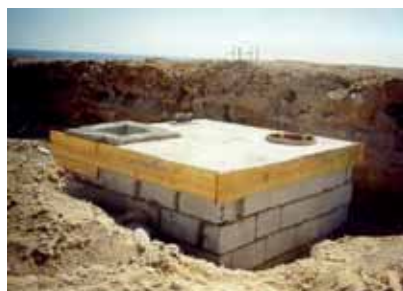
However small the flow of sewage, it must never be tipped directly. Thus, cesspits or portable treatment plants are installed in FCC's projects, with the relevant authorisation and with period analyses of the quality of the outlet.
