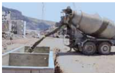
The rational use of water is an elemental practice that is simple to apply. The idea is not to skimp on its consumption but to consume strictly the amount that is necessary. This is achieved, for example, with techniques such as the re-use of water for washing conduits.
