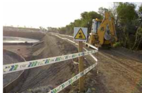
The delimiting of areas of access and occupation is important, signposting the entrance and exit for vehicles in the project and external to it. Preferably, existing tracks are used before new ones are created and in cases in which this is not possible, they are created so that they cause the minimum visual impact and so that they may have an alternative use in the future, as a forest track, for example.
