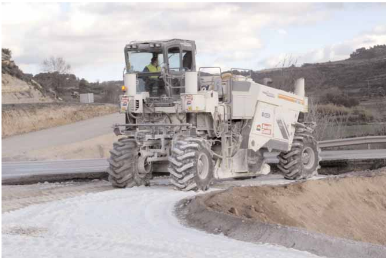
The stabilisation of land with the use of lime or cement prevents the need for removing it, thus reducing the amount of waste generated and the need to consume resources, optimising their management.
