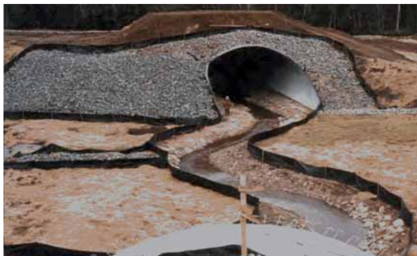
When necessary, filtering barriers are used to protect watercourses from surface run off, preventing the transport of fine material from the environment and an increase in the water's turbidity.
