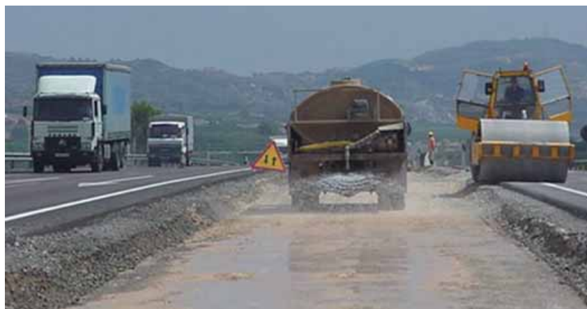
A simple but extraordinarily effective measure to control dust emissions generated by moving machinery is to spray tracks and stockpiles, which can be reinforced with the addition of agents or hygroscopic salts to increase its effectiveness.
