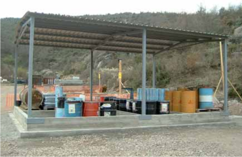
The arrangement of tubs, preferably compartmented, for storing dangerous substances and products centralises their storage in a single point and prevents their accidental tipping or spilling.
