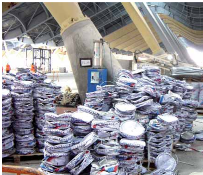
The use of means to compact wastes generated (in case of the photograph, paint cans) reduces the space occupied by them and the volume to be transported. This means that the transport of the waste is much more efficient and the associated financial and environment costs are minimised.
