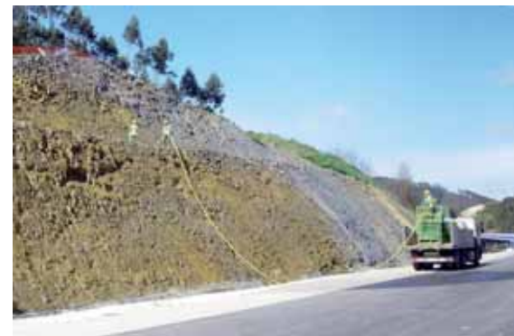
Operations such as hydro seeding allow the restoration of areas whose environmental value may have been reduced by the project's installations and activities, adapting the affected terrain whose shape and landscape has been affected and integrating it into the surrounding environment.
