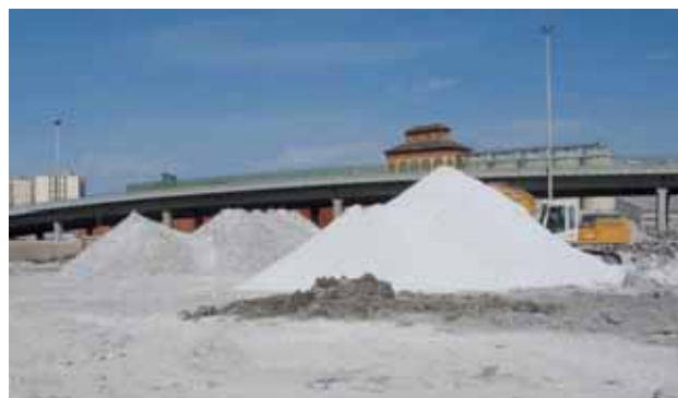
One of the good practices adopted by FCC Construcción in the area of wastes is the valuing of rubble from demolition to form gravel which is used as a new raw material.
