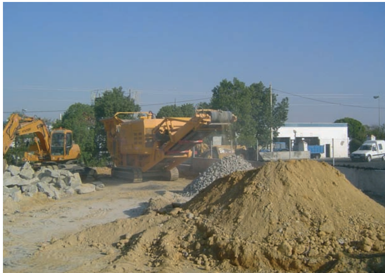
Materials from excavation on the site itself or from other, nearby sites can be treated and made use of, reducing consumption and the generation of tips
