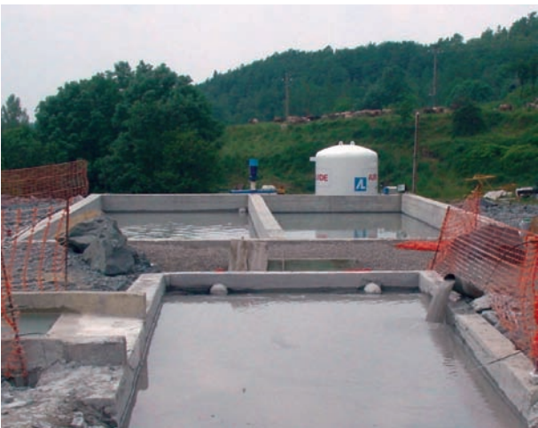
The waste output is initially decanted before passing to neutralisation ponds using carbon dioxide at the exit from the tunnel, removing suspended solids and reducing the pH
