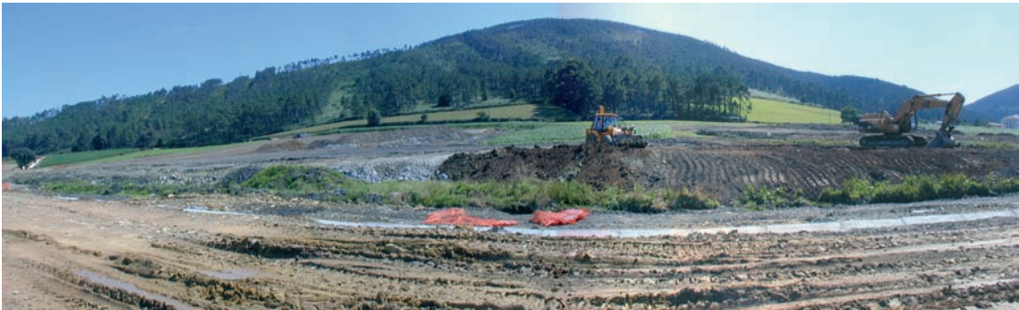
Topsoil is a scarce and valuable resource which we must try to re-use on the sites themselves. Excesses must not be tipped but used on the site or to improve nearby land
