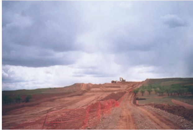
Increased distances in the masses diagram to compensate for earth in embankments and cuttings allows great savings in loans and important economies in tipping
