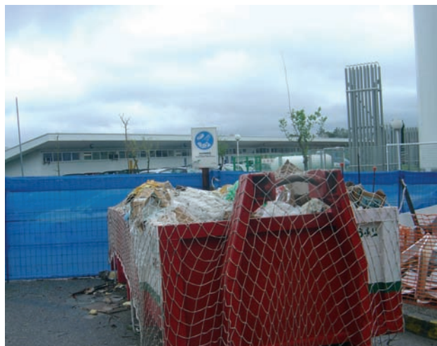
Clear signposting of containers, the protection of their contents from being scattered by the wind and a suitable classifying by categories, allow their better and more effective use
