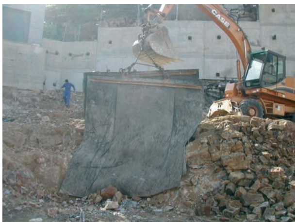
Blankets placed on the surface when blasting prevent flying material and the generation of dust
