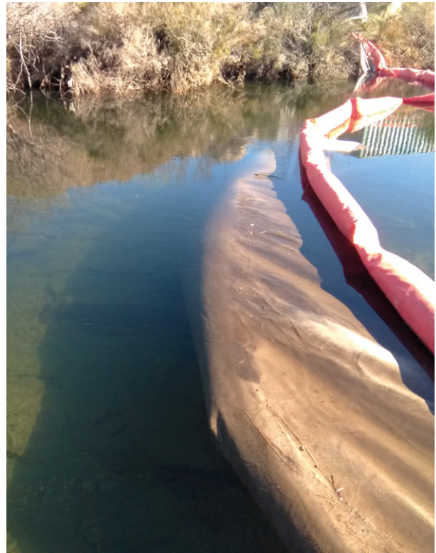
This barrier consists of a floating part and another anchored to the riverbed, which retains the cloudy water and filters it.
