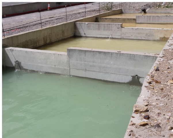
The use of these ponds makes it possible for suspended solids to be deposited before the water is discharged into the river.
