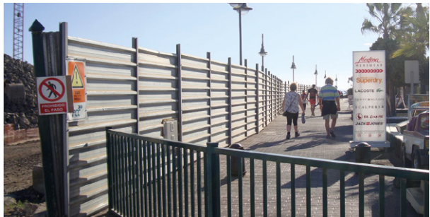
The barrier set up along the perimeter of the worksite acts as an acoustic buffer.
