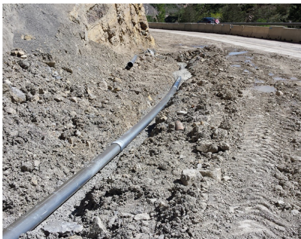
The discharge generated by drilling and upwelling was diverted to the settling ponds.
