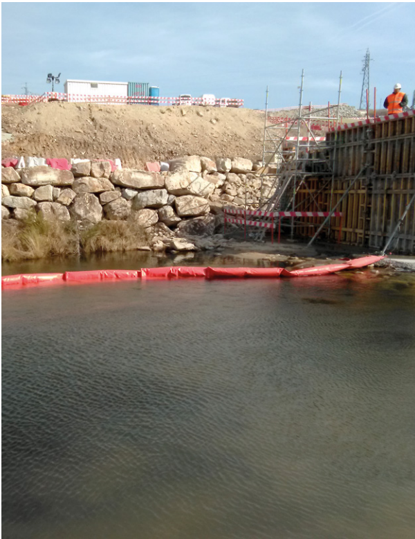
The geotextile barrier retains particulate matter around the worksite.
