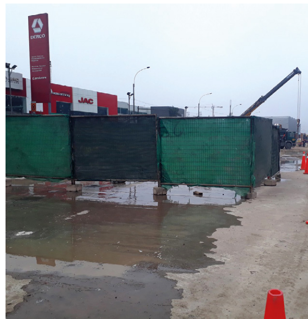
The mesh is easily positioned depending on the direction of the wind to prevent the dispersion of particles.
