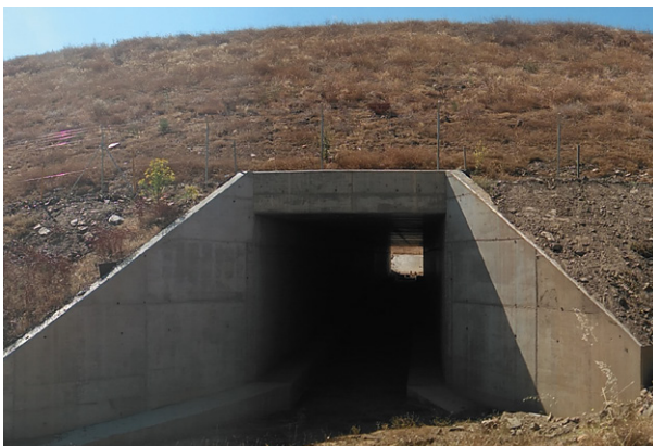
Cross-sectional drainage work prepared as passage for wildlife.
