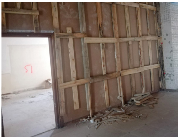
Frame that supports the geotextile protection for the part of the mural that remained on the building.
