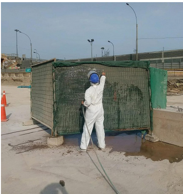
An operator dampens the raschel mesh around the concrete cutting area.
