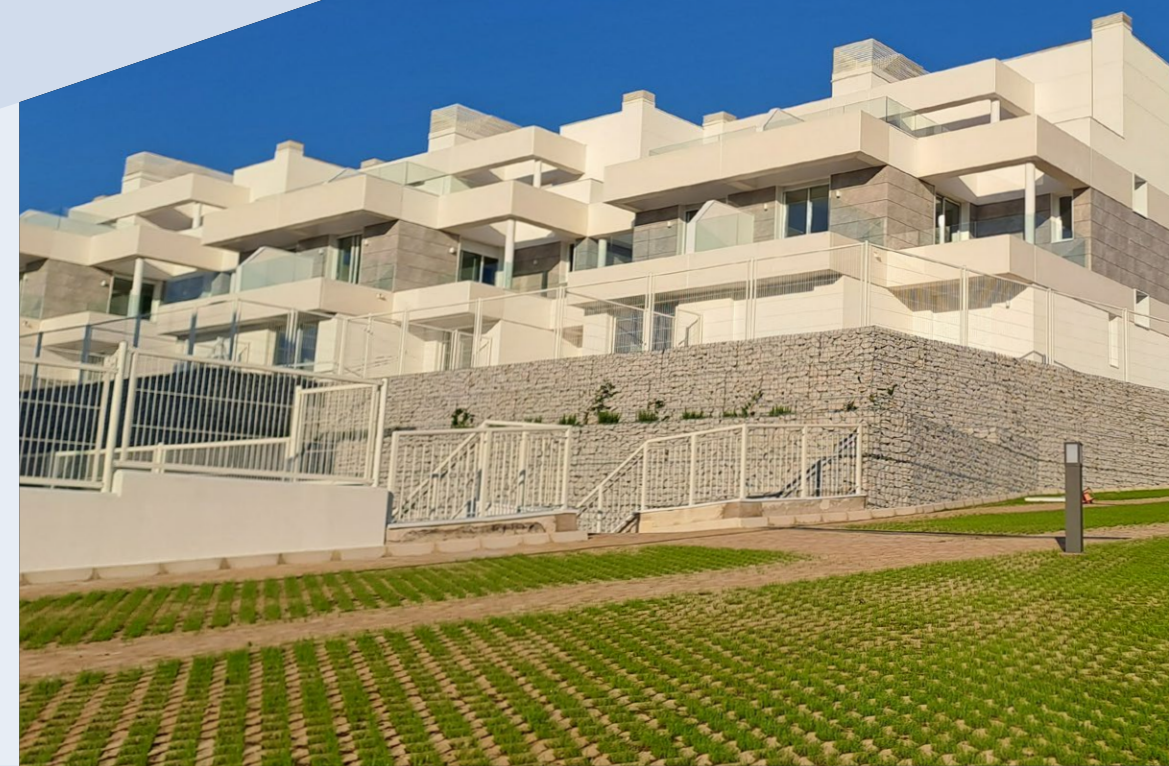
Housing in Arroyofresno. Madrid, Spain.
