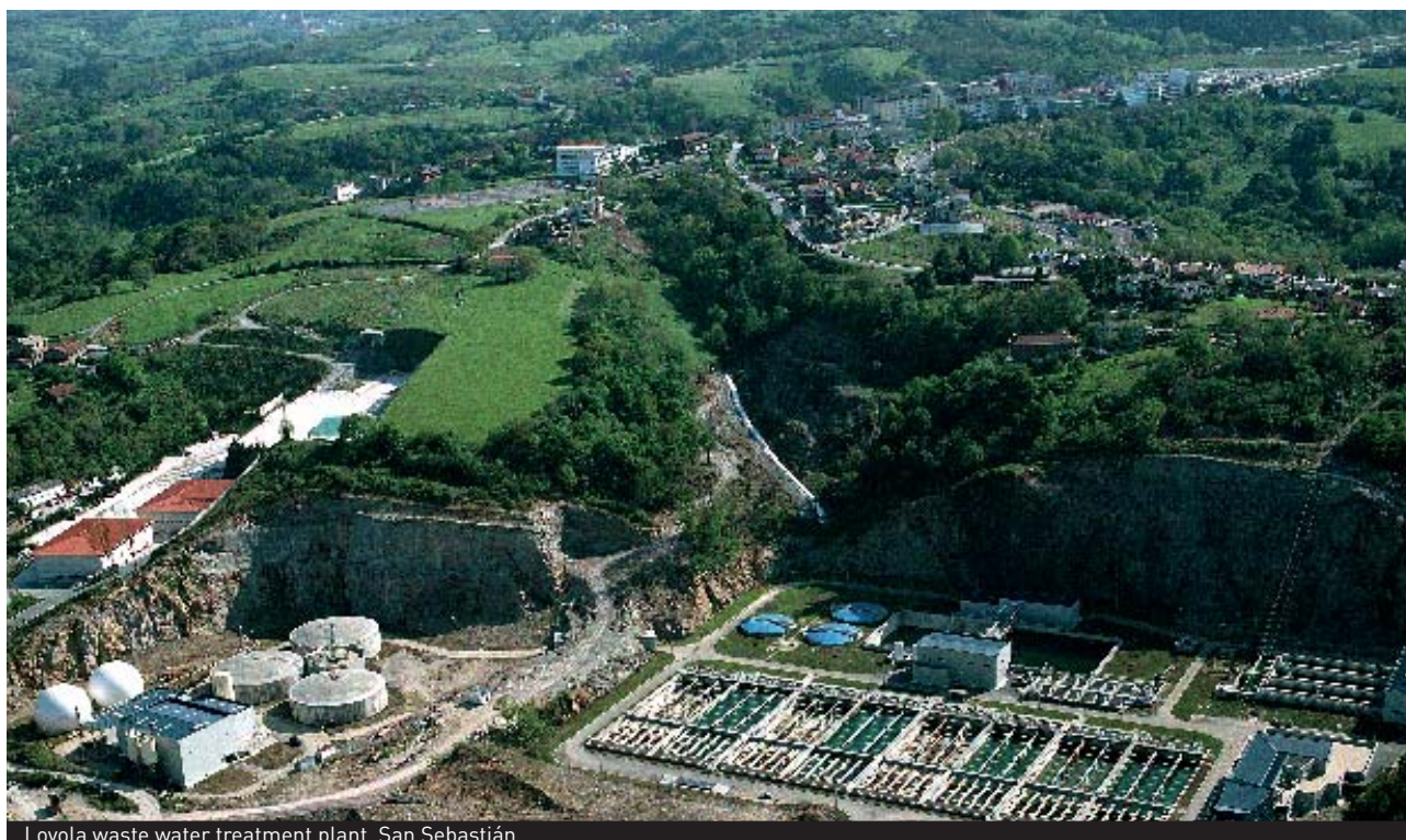
Loyola waste water treatment plant, San Sebastián
