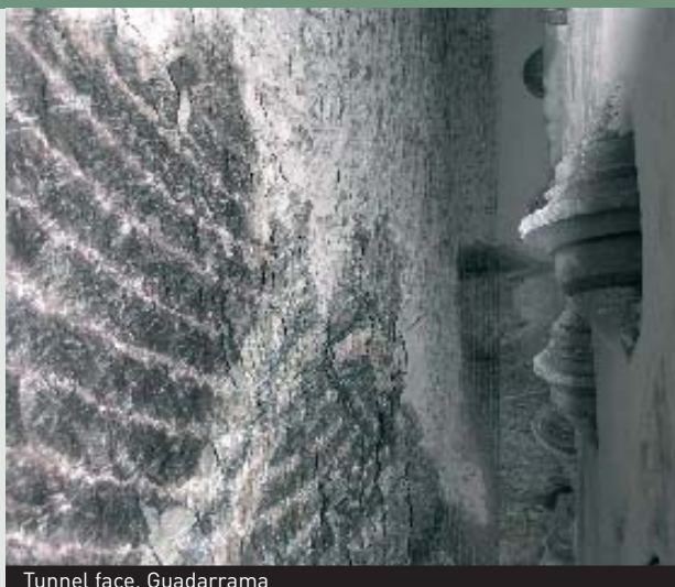
Tunnel face, Guadarrama
