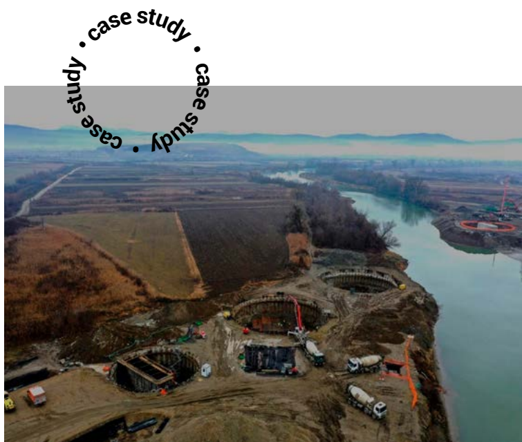
Sheet-pile enclosure for the bridge over the Mures river (Romania)
