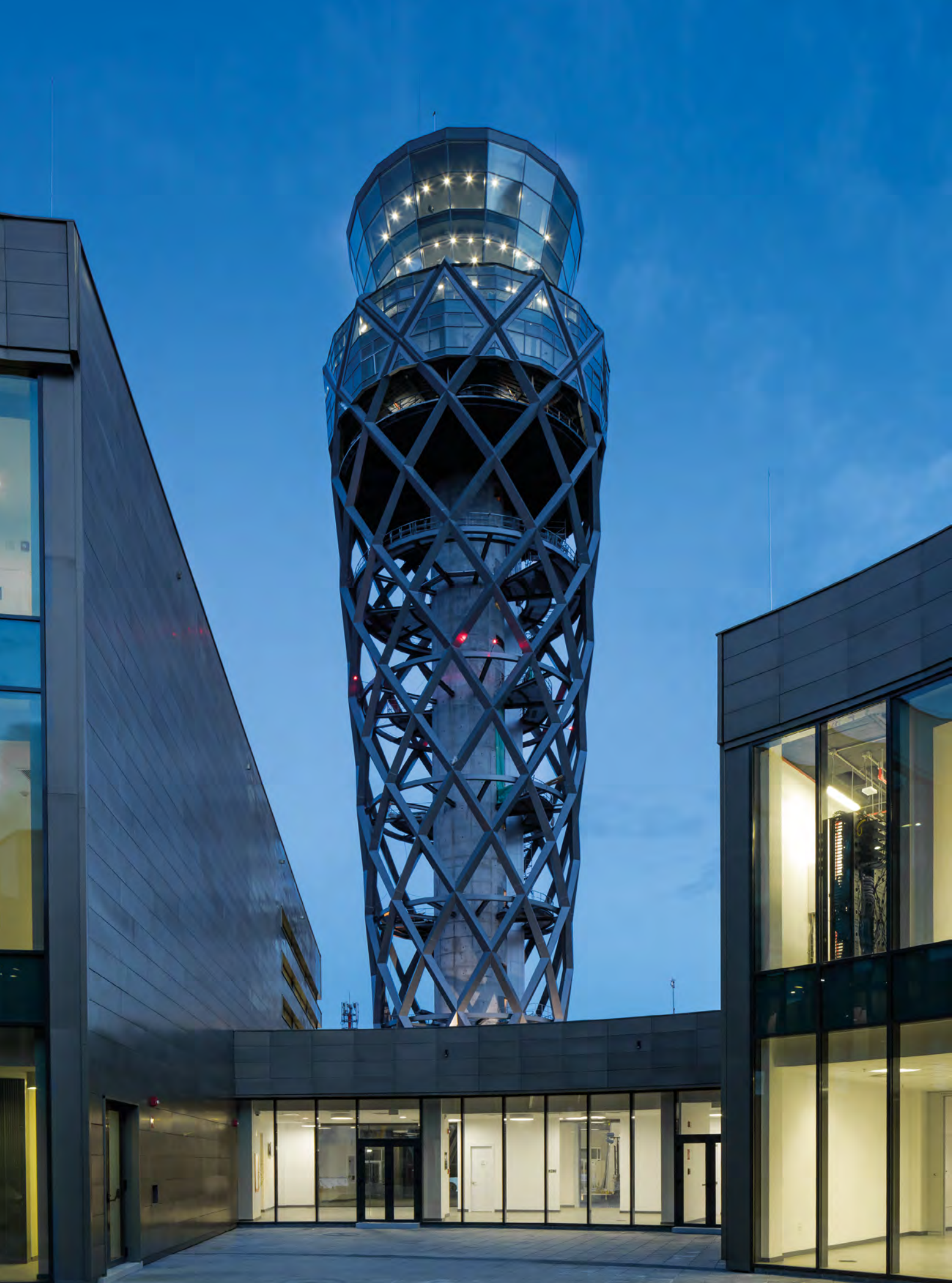
Control tower of El Dorado's airport, Colombia
