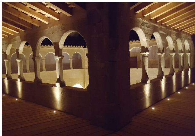
Rehabilitation of the Riudeperes monastery, Catalonia, Spain.
