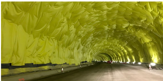
Coating of the Vallirana Tunnel, Catalonia, Spain.
