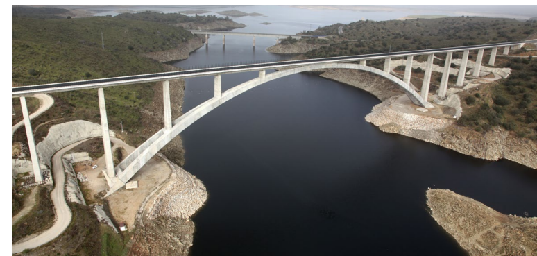
Viaduct of Almonte. Ave Madrid-Extremadura, Spain
