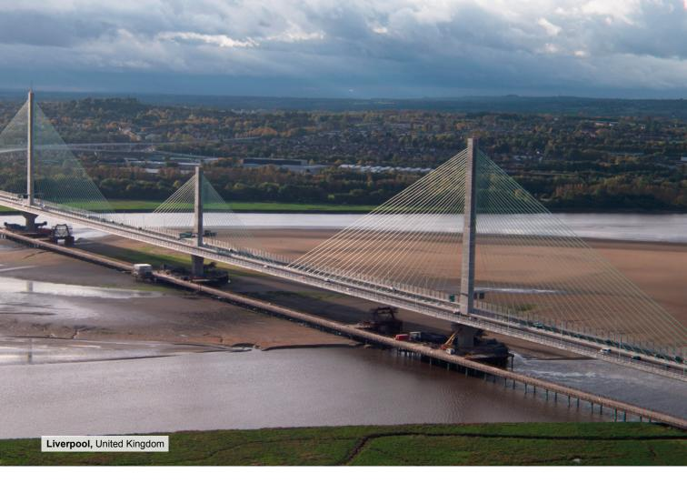
Mersey Bridge The project included design, construction, financing, maintenance and operation of the bridge over the Mersey River (United Kingdom). The 2,250 meters long bridge includes three central cable stayed spans that go up to 318 meters. The width of the deck is variable at up to 43 meters.
