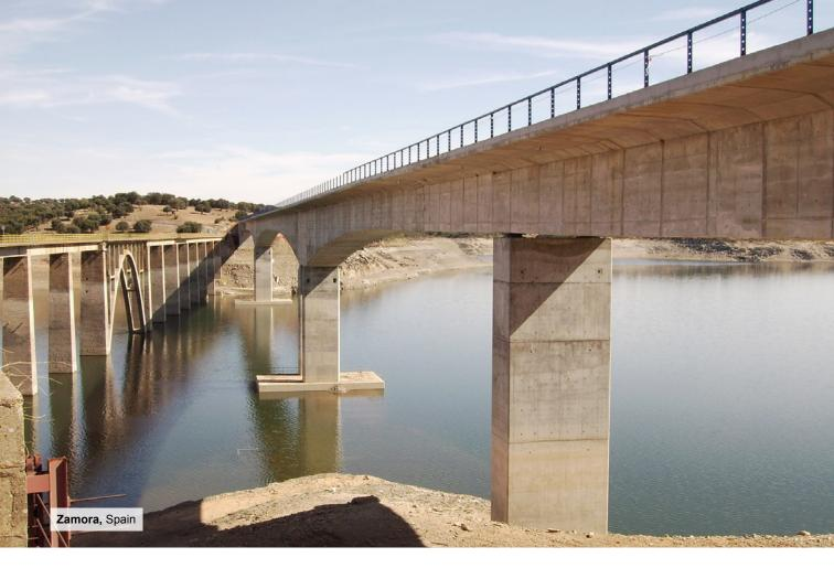
**Ricobayo** Reservoir <sub>Viaduct</sub> This pre-stressed, concrete bridge has the longest span of 155 meters, which is also the longest high speed railway span in Europe. The bridge was constructed using cantilevered advances with cast in-situ segments.
