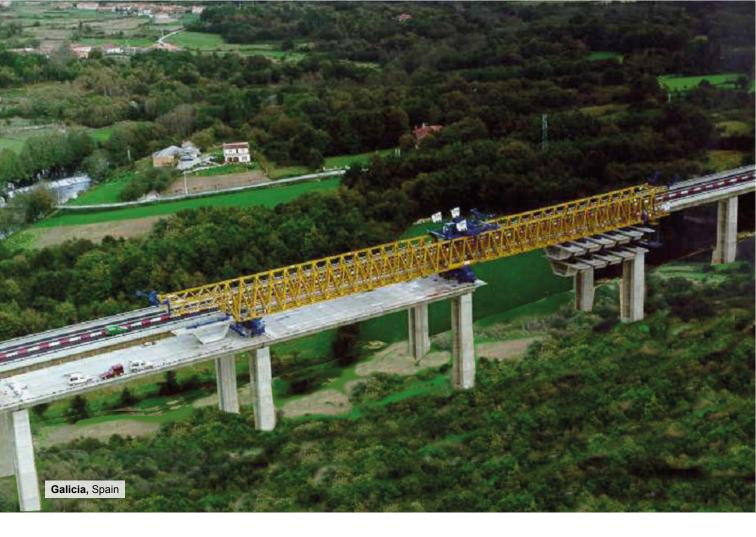
Arnoia and Valenzana Viaduct These viaducts are located on the Rías Bajas highway (Galicia), on the stretch San Ciprián de Viñas - Alto de Allariz. The Arnoi and Valenzana viaducts are 945 meters and 450 meters long respectively. The sections are erected isostatically to bridge to construct the 45 meters spans with 16 prefabricated, pre-stressed segments.
