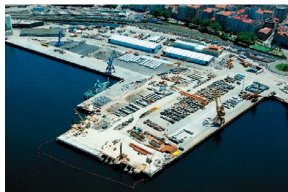
● The silt barriers impede dispersion of fine emulsion and other substances such as oils or hydrocarbons. Thus the surrounding waters are protected from pollution.
