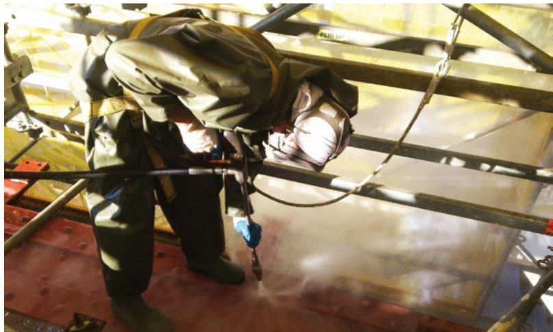
Washing the viaduct's steel structure.
