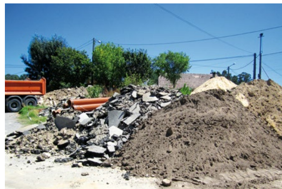
● One of the main challenges we face in our projects is the reduction of resources used and waste taken to landfills. One way of reducing this is reusing construction waste as filling material, thereby reducing the amount of loaned soil.
