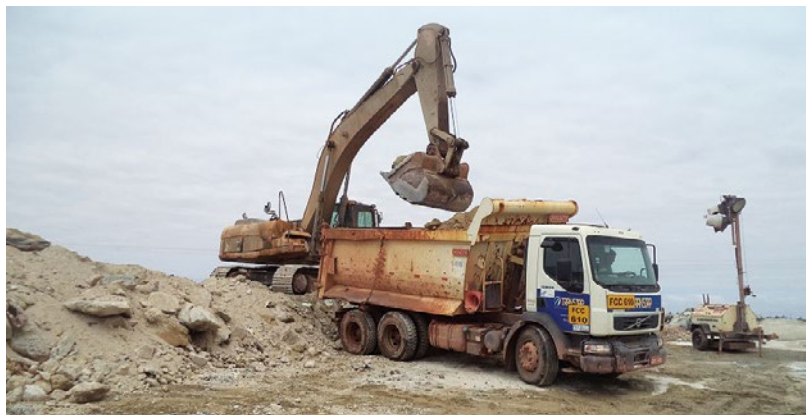
Preparation of waste material with hammer head excavator.
