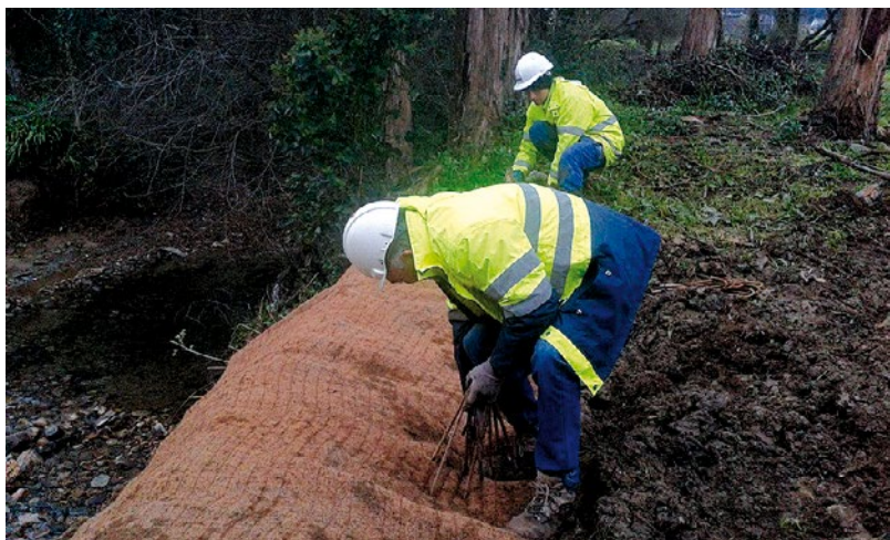
Barrier between flood areas and stretch of pipeline.
