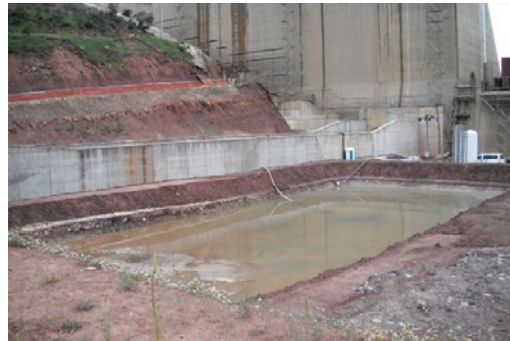
Control unit for monitoring pH, regulating influx of CO 2 and catchment pool for subsequent treatment with CO 2 .
