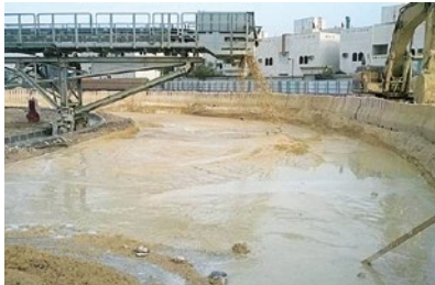
Collection of material extracted from tunnel boring machines in line 5.
