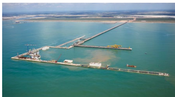
● Construction of a breakwater at Puerto Açú, Río de Janeiro (Brazil)
